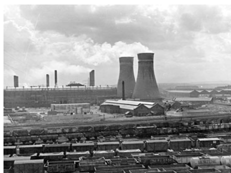
Blackburn Meadows Power Station courtesy Sheffield Local Studies Library
